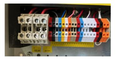
Full set of Connecting Terminals For battery, solar, Safety devices, keypads, CXN Bus Devices, battery cabinet alarm, Earthling rod connection & Battery backup connections
